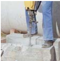
Breaking Concrete
